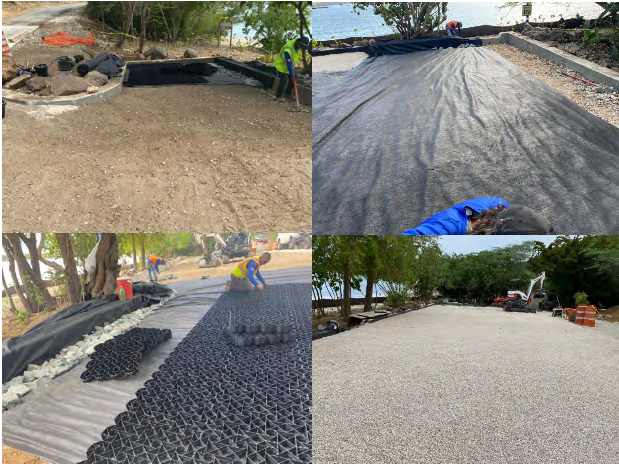
Figure 5. The process of developing the permeable parking lot at Tamarindo Beach.
