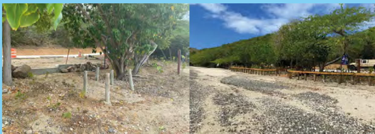
Figure 47: Previously installed and damaged wooden poles (left) have been removed and replaced with new wooden poles and wooden sidewalks (right). (Source: PDC)
