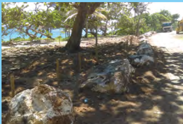
Figure 28: Laying boulders to prevent car traffic on the beach (Source: Adam Gibaud (ONF); 10/22/2020)
