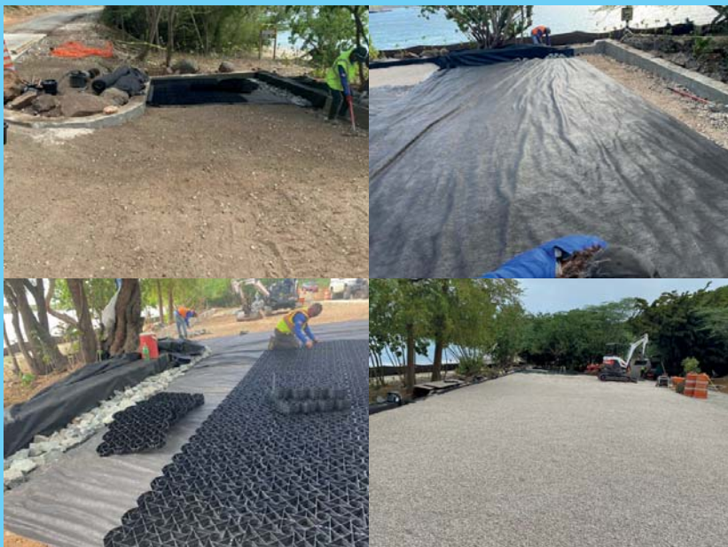
Figure 46: Tamarindo Beach Permeable Parking Development Process (Source: PDC)
